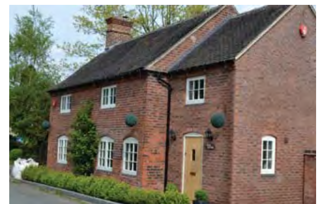
Window detail: painted sash with curved brick arch to top
