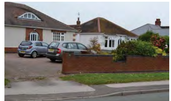
1.5 storey rendered dwelling with curved brick detail above window.
