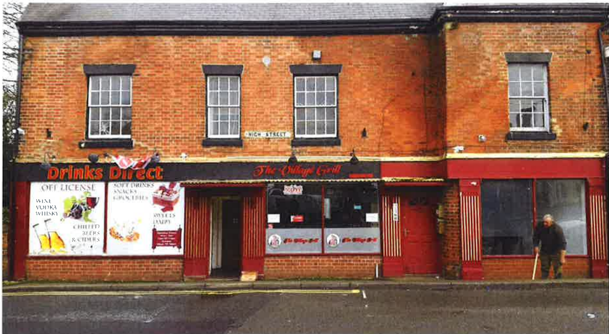
Current view of the building.
