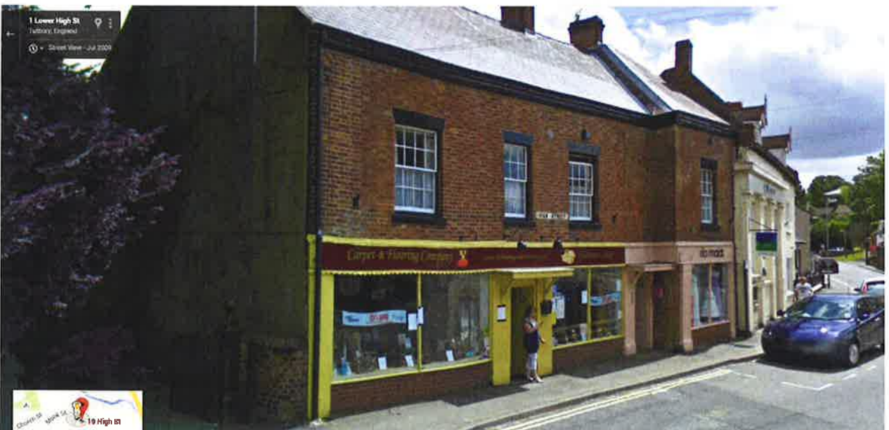
View of the building taken in 2011.
