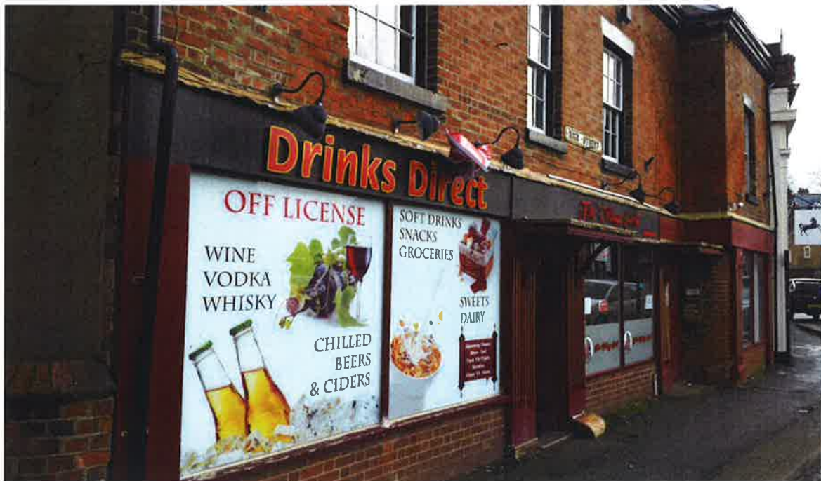
Current view of the building.
