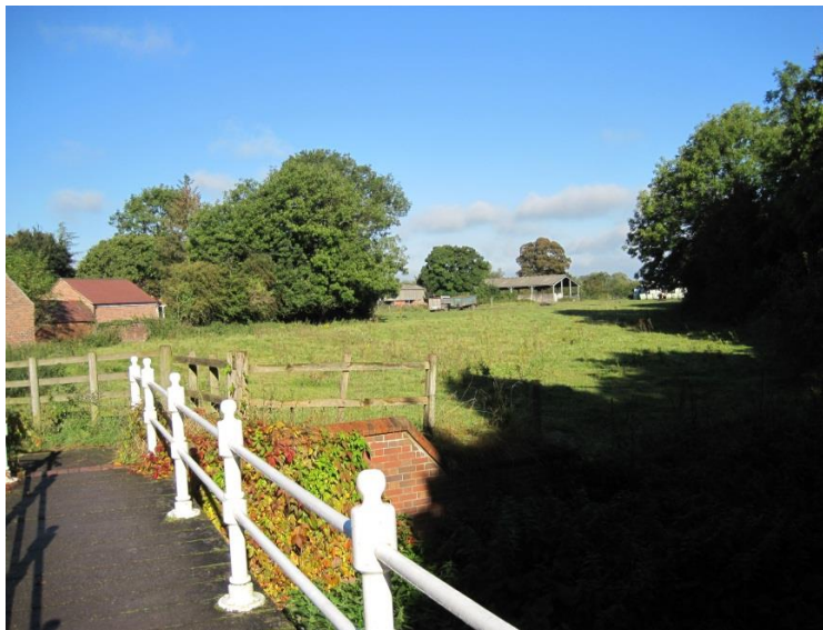
Figure 18: View from the bridge at the Brookhouse
