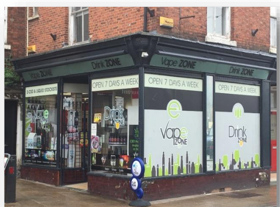
Above: While the elements of the shopfront reflect traditional design the use of extensive signage and vinyls detract from this and deaden the frontage which erodes its character.
