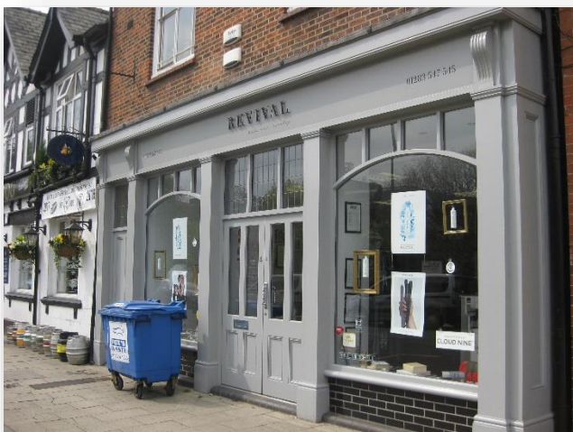
Left: A new shopfront that references traditional design. The elements of stallriser, pilaster, corbel, fascia and cornice are all evident with elements that present a more contemporary twist e.g. the glazed black brick stallriser and arched clerestory.
