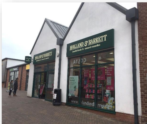
Above: A modern shopfront that reflects the typical characteristics of shopfront design with mullion and transom details that breaks up the glazing and adds verticality to the design.
