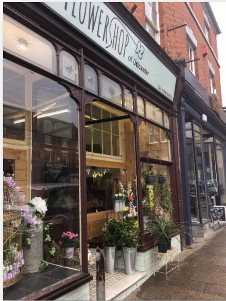
Above: Traditional shopfront with clerestory with decorative frosted glazing and spandrel detail (bracket at the corner of the windows). This helps in breaking up the extent of glazing.
