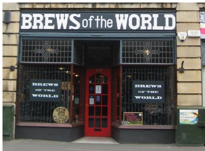
Right: A more discreet design of security measures with bars placed behind the glazing which also allows for views into the shop. These should be removed during operational hours to present a more active frontage.
