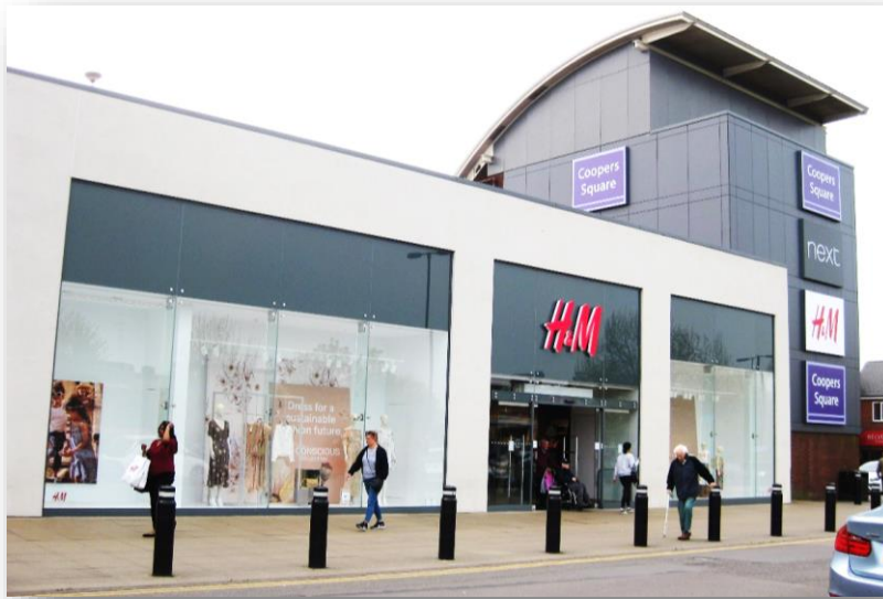
Above: A contemporary approach to shopfront design with a large extent of glazing that provides a large display area and results in a more lightweight character. The different colour division at the top provides a clerestory and fascia for signage.
