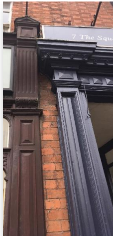
Timber pilasters with different relief detail and corbel/console detail.
