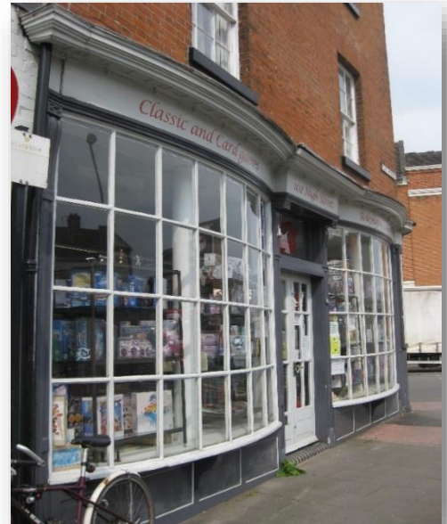
Above: A different type of shopfront with bay windows and glazing bars that reflect the Georgian character of the property.
