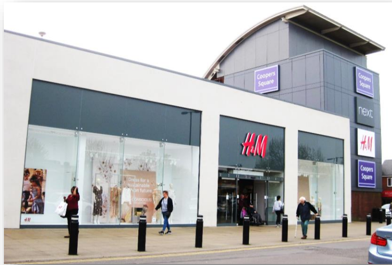
Above: A contemporary approach to shopfront design with a large extent of glazing that provides a large display area and results in a more lightweight character. The different colour division at the top provides a clerestory and fascia for signage.
