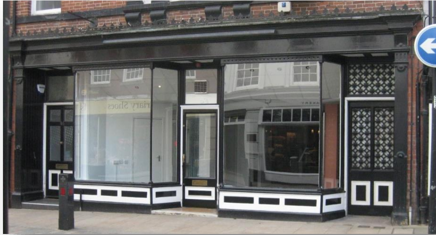
Above: A typical traditional timber stallriser which helps ground and protect the shopfront. The height of the stallriser carries through to the door panel.
