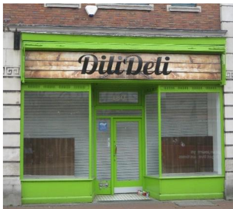
Left: Despite displaying all the elements of a traditional shopfront the garish colour finish detracts from this and fails to respond to the building or its setting.
