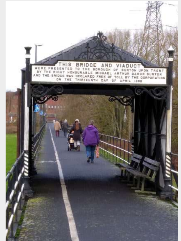
Photograph of the existing Ferry Bridge across the River Trent at the south of the town. Project F proposes a new cycle and footbridge at a more sustainable height level than the Ferry Bridge.
